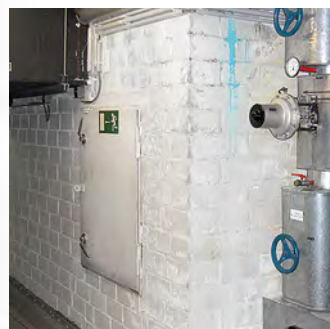
Uranin Blue is extremely luminous under UV light and, due to its good capillary flow, is ideal for leak detection when mineral building materials needs to be penetrated.
