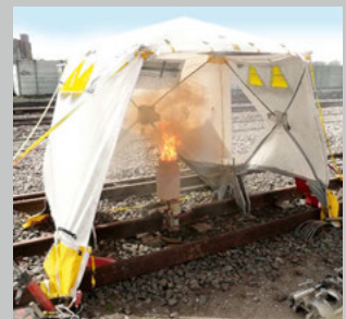
TRACK CONSTRUCTION WORK TENTS for welding work
